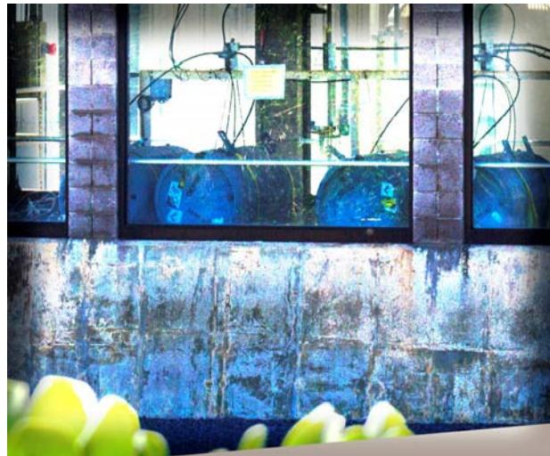
Chlorine tanks strapped to floor 3/11/11. Note apparent tsunami water height mark on exterior concrete blocks.
